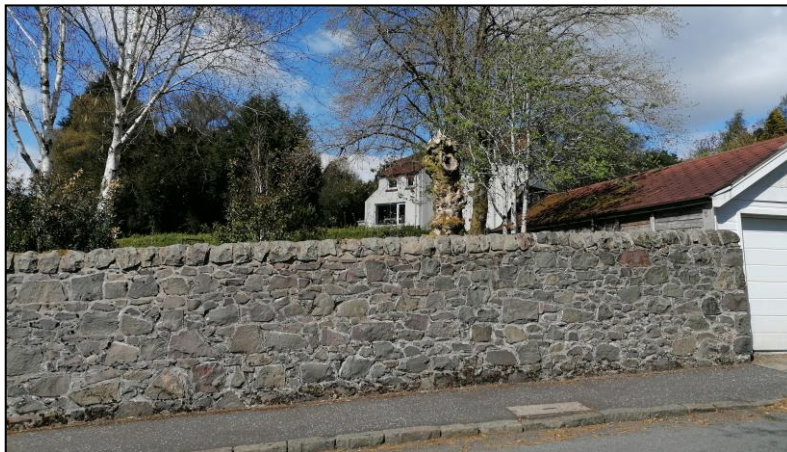
Site as viewed from Houston Road
